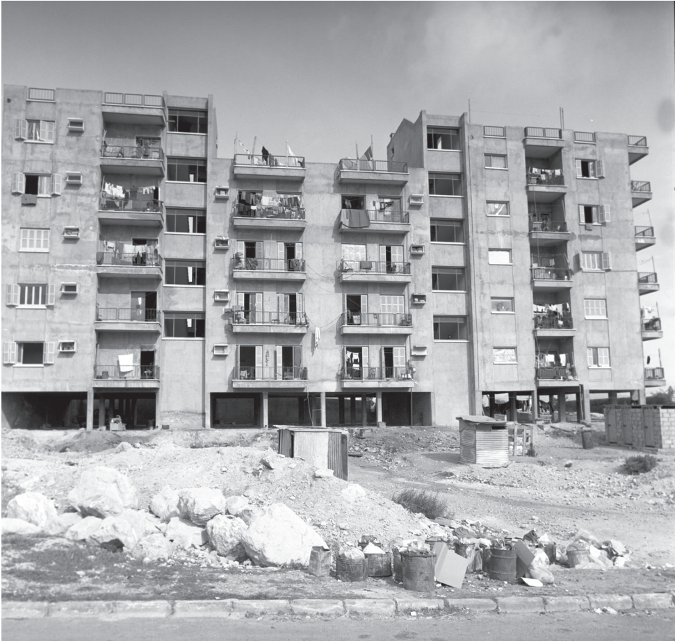
Photo 4. Completion of blocks of flats, Strovolos
