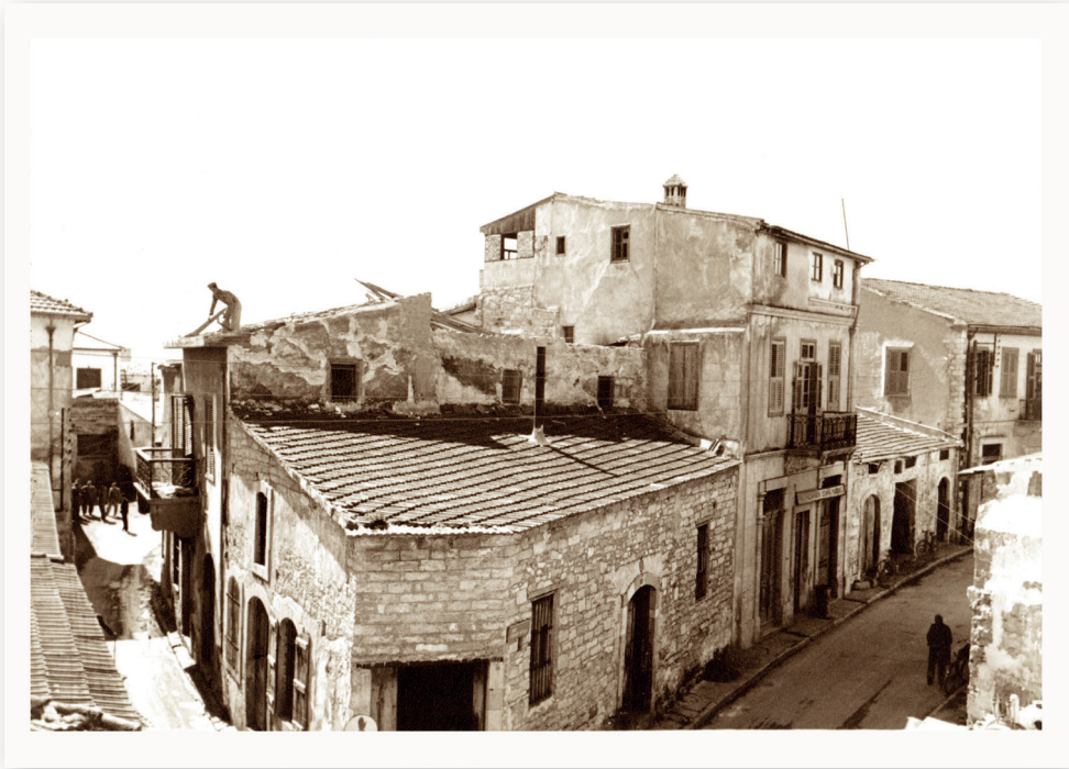
Zig-Zag Street, Limassol.
